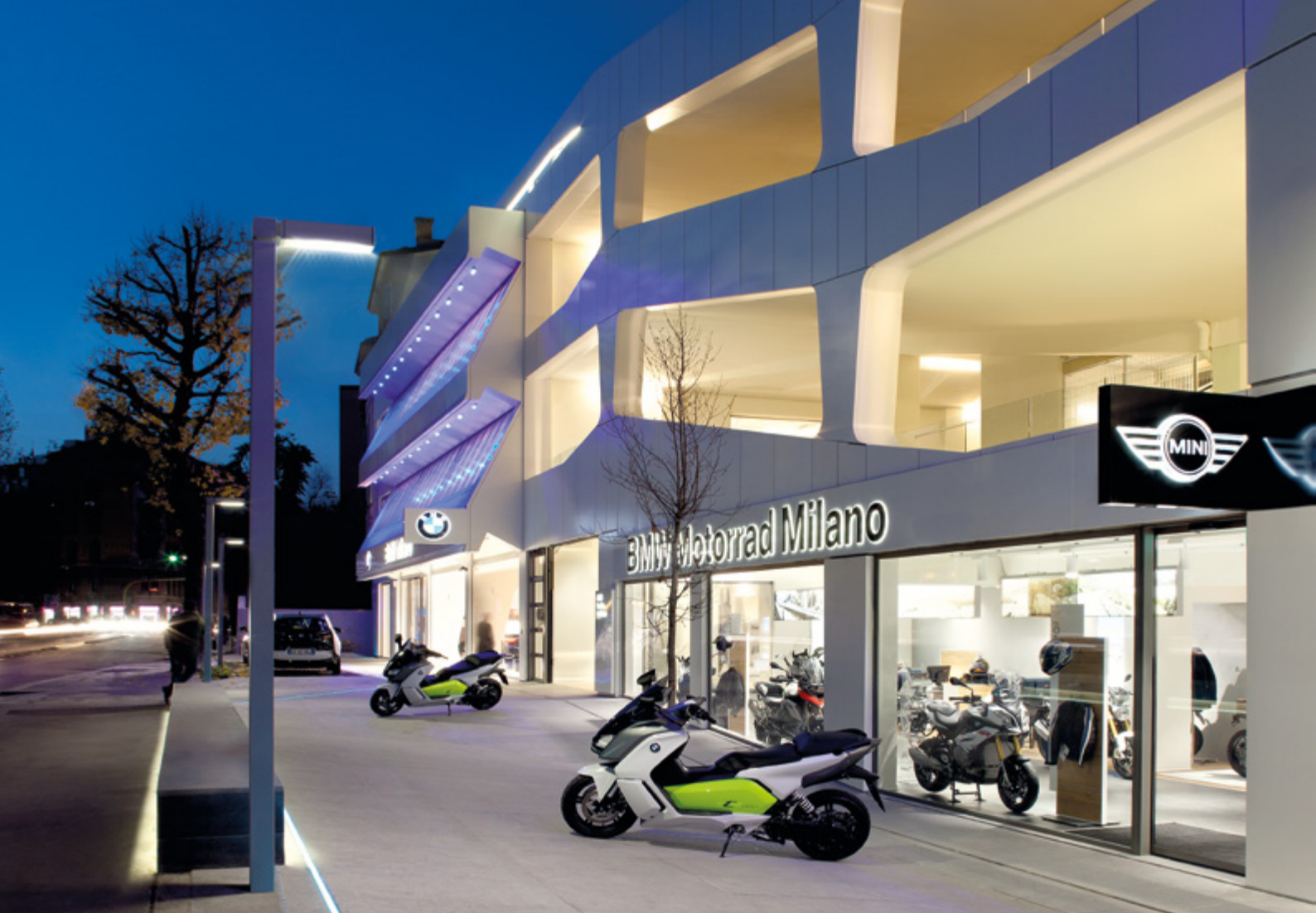
BMW Milan City Sales Outlet Via De Amicis, Milano, Italy / General contractor: ISG Italia © Ph. Barbara Corsico
